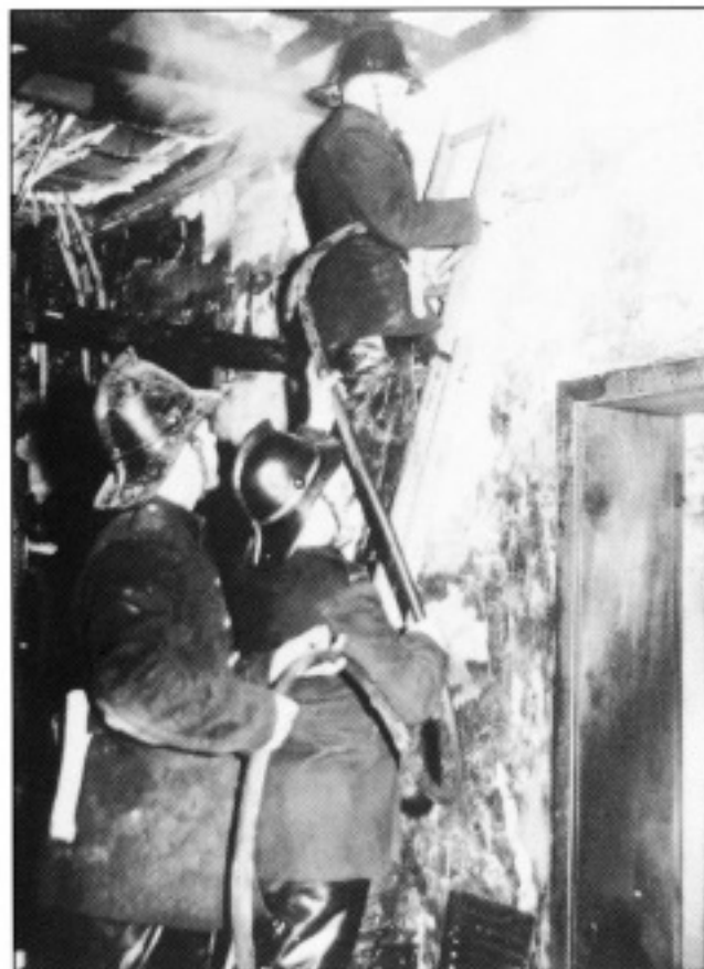
Left: A calamity at Newcastle! A major fire damaged the hostel but Fellowship members rallied round and residents were found accommodation locally and Christmas card distribution was only slightly affected.
